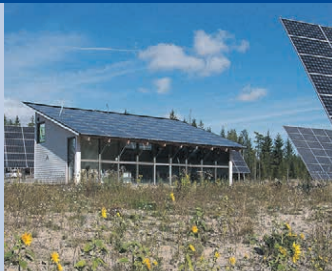
Fig. 2 - Sunflowers and part of the 1 MW PV installation outside of Västerås. A recently published monitoring project has compared the output from fixed, 1-axis and 2-axis tracking systems, with and without power optimizers (Photo: Bengt Stridh).
