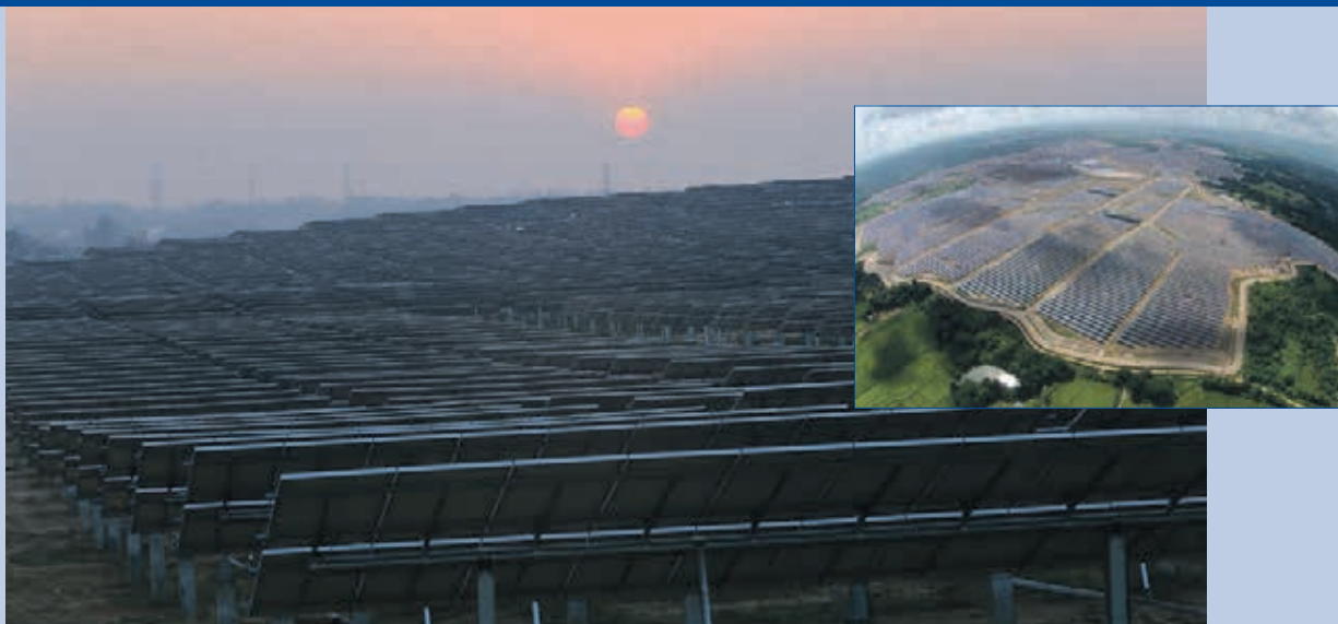
Fig. 3 - The Biggest SPP Project in 2015. This project has achieved COD since February 2015 in Lampang province. Total installed capacity 126,396 MWp with Poly Crystalline Solar Cell, Solar Tracking System (Photos: Energy Absolute Public Company Limited).
