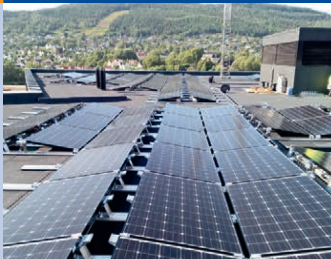
Fig. 2 – Omsorgsbygg Oslo installed a 130 kWp system at Økern Sykehjem (a home for elderly people). The power from the system is for self-consumption (Photo: Fusen AS).
