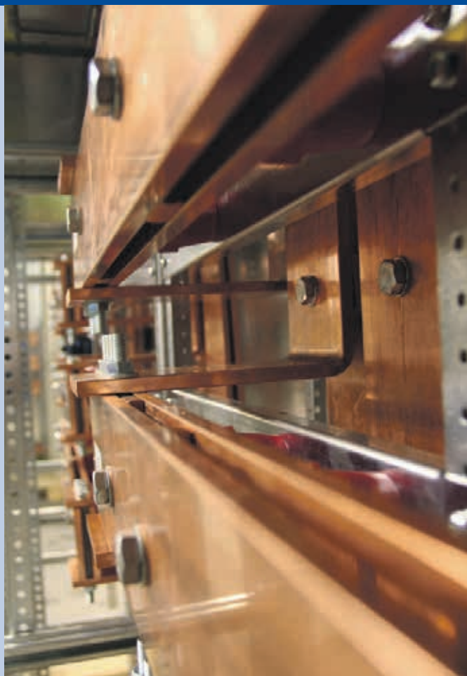
Fig. 1 – Copper busbars.
