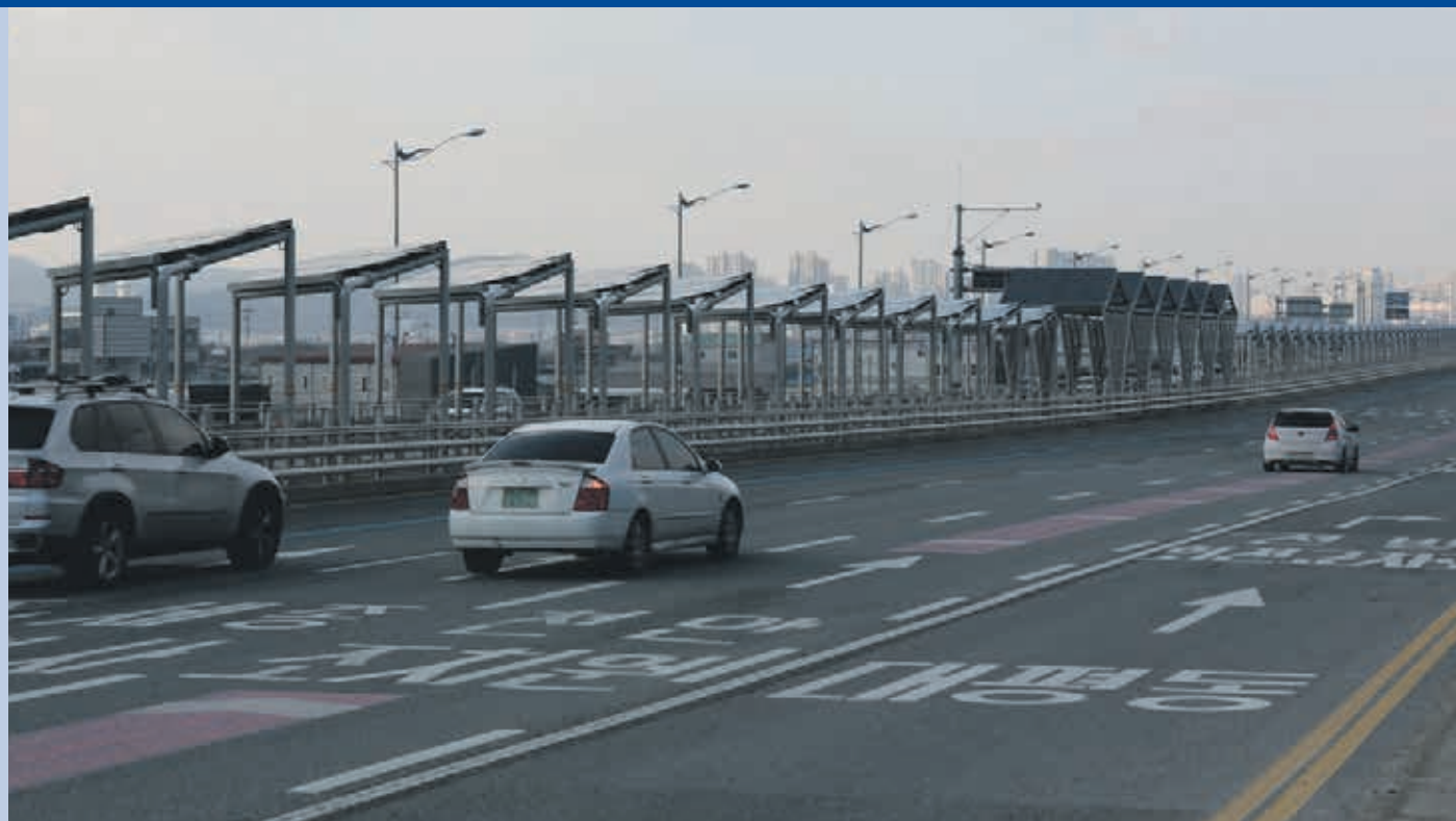
Fig. 1 - Bicycle lane covered with solar panels, Sejong-si, Korea.
