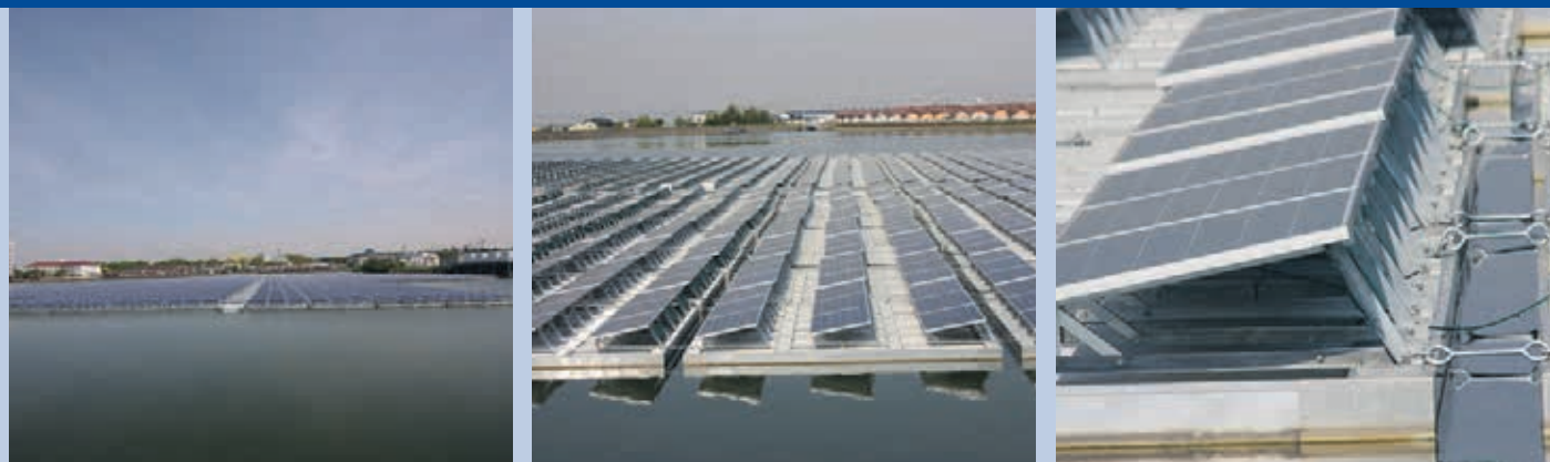
Fig. 1 - Floating PV Power Plant (INFINI Hyogo Daikyu Power Plant) (Inami Town, Hyogo Prefecture). Multicrystalline silicon PV module: 250 W x 6 846 modules (by INFINI) 1,7 MW.
