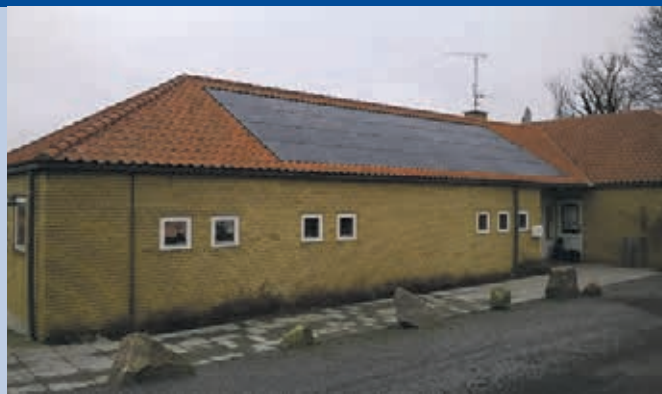
Fig. 4 - Roof integrated PV system by Storløkke holiday centre in Bornholm. A part of the PV Island Bornholm R&D project. Developed by Nielsen EI, Rønne.
