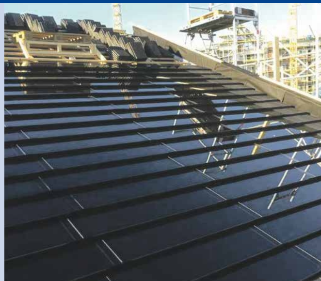
Fig. 3 - PV integrated roof tiles by Soltech Energy on a residential building in Linköping (Photo: Soltech Energy Sweden AB).
