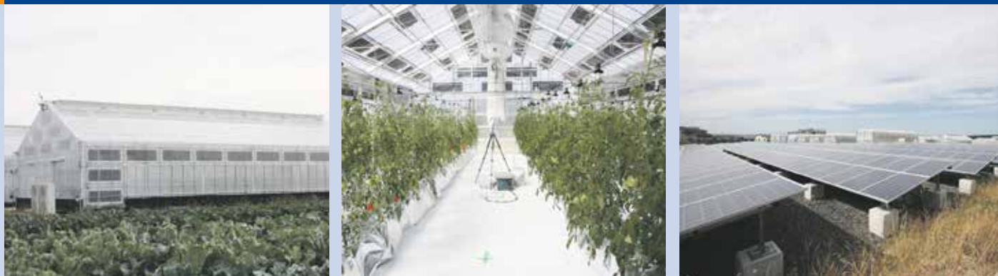
Fig. 2 - PV System on the Farm of the Graduate School of Agriculture, Kyoto University (Kizugawa City, Kyoto Prefecture). PV system on a plastic greenhouse: 2.15 kW, Organic thin-film PV module (by Mitsubishi Chemical, 25 W x 86 modules). Ground-mounted PV system: ca. 400 kW, Crystalline silicon PV modules (by Toshiba).
