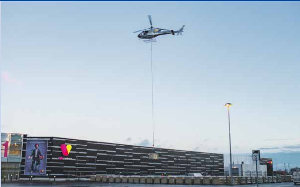
Fig. 1 - A helicopter lifting PV modules while constructing 1,1 MW rooftop system on Väla centrum, Helsingborg (Photo: Niklas Lydeen).
