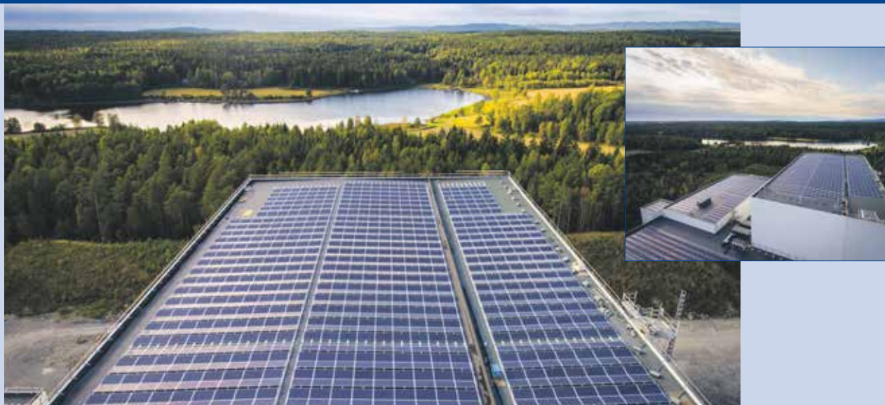
Fig. 1 - 1322 kW rooftop/wall PV system installed in 2016 at UNIL's distribution center in Våler, Norway. (Photo: Leif Skorge, MultiConsult AS).
