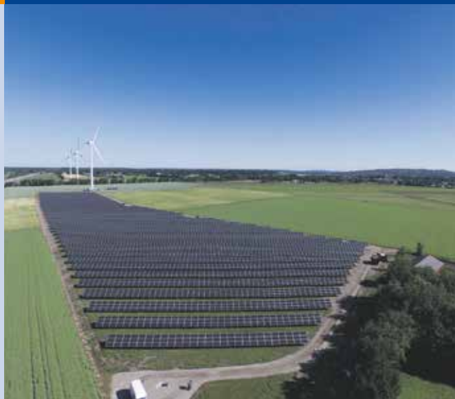
Fig. 2 - The new PV power plant "Solsidan" in Varberg (2,7 MW) can reduce electricity connection costs thanks to co-location with wind turbines (Photo: Solkompaniet).
