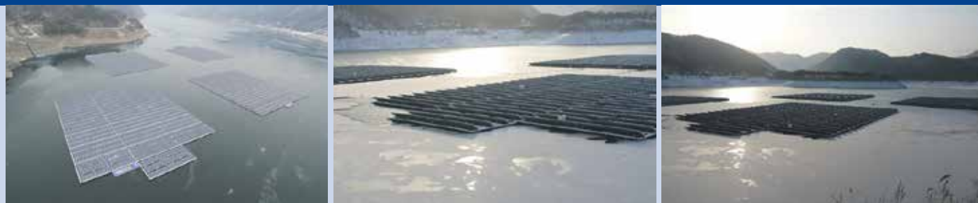
Fig. 1 – 2 MW Floating PV system at Boryeong Dam, Boryeong-si, Chungcheongnam-do, Korea.
