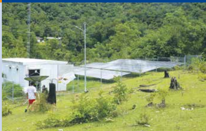
Fig. 6 – 20kWp PV village supply system, Gajah Bertalut, Riau, Sumatra, 2016 (Photo: Fraunhofer ISE).
