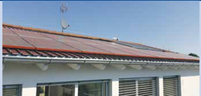
Fig. 2 - Roof integrated 4,5 kW PV plant at Solferino (MN), Polycrystalline modules with red cells and frame (Photo: Solmonte www.solmonte.it ).
