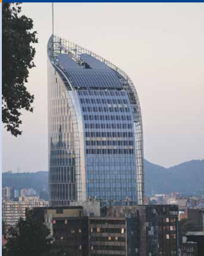
Fig. 2 – Issol installed 126 kWp on the new Federal Finance Tower in Liège. They have developed glass-glass PV modules with a limited thickness of 10 mm. This installation will produce approximately 100 MWh per year.
