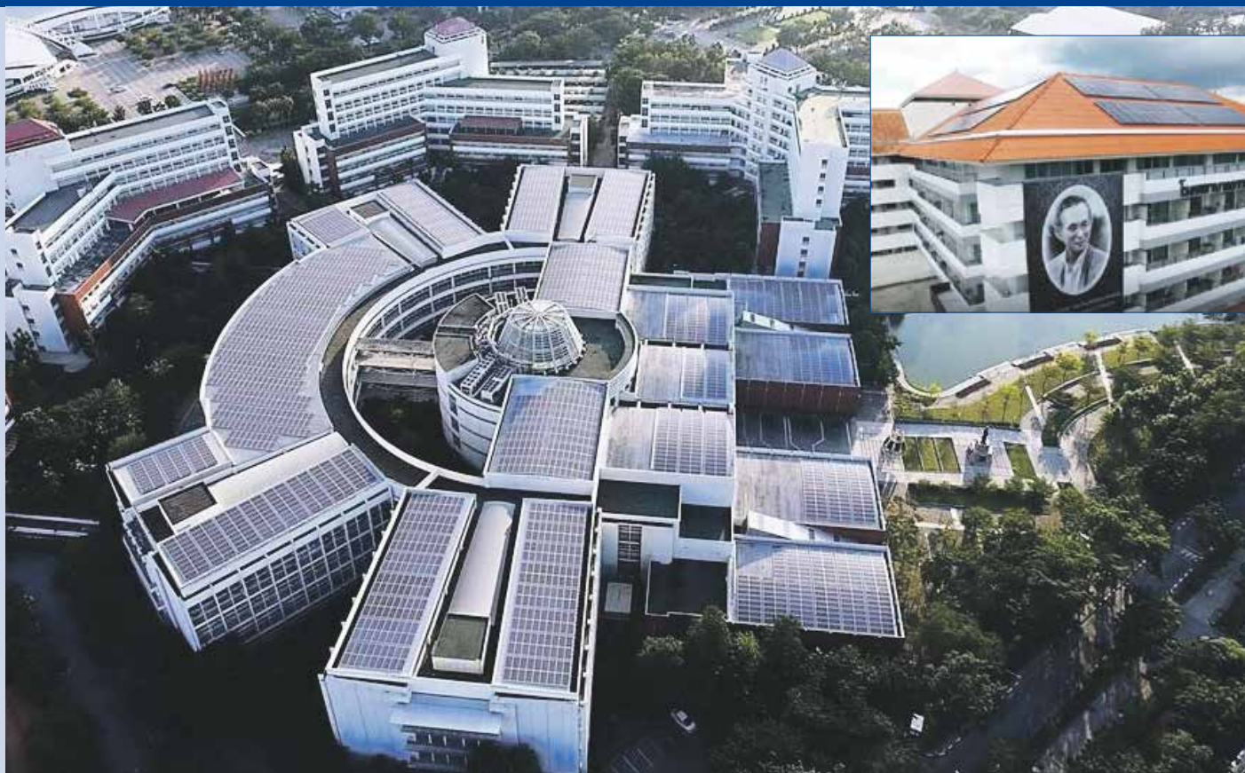
Fig. 1 - The solar rooftop at Thammasat University is the biggest solar rooftop of the University in Asia. The total installation target is 15 MW in 2016 (2015: 6 MW, 2016: 9 MW) (Photo: Solartron Public Company Limited).
