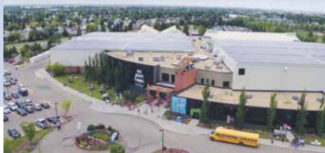
Fig. 2 - The Leduc Recreation Centre PV system, located in Leduc, Alberta, has 3 622 solar PV modules for a total capacity of 1,14 MW. It is the 2 nd biggest roof-top PV system in the country, generating approximately 15 % of the centre's annual energy consumption and saving the city some 90 000 CAD each year.
