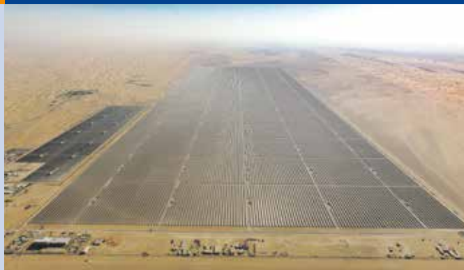
Fig. 8 - Mohammed bin Rashid Al Maktoum Solar Park, Dubai (UAE) - Phase II, built by Spanish TSK Company. 260 MW photovoltaic plant. Type of module: CdTe. Fixed supporting structure.
