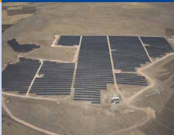
Fig. 1 - One of the two PV power plants in the licensed segment in Elazığ (8 MW) [15].
