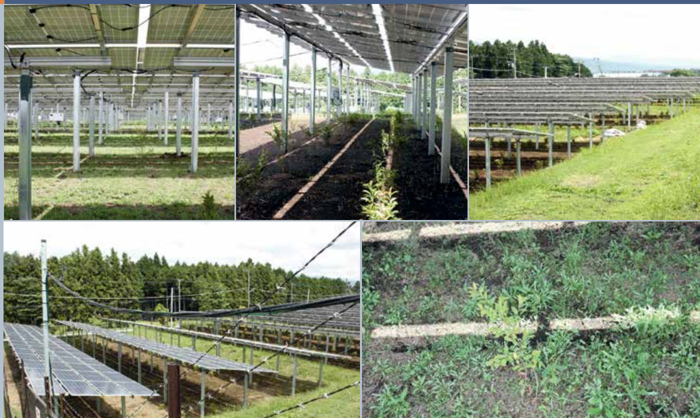
Fig. 2 – Large-scale PV systems on farmland (Gotemba PV Power Plant No. 1 & No. 2) (Gotemba City, Shizuoka Prefecture). "SPLITMAX" PV modules using half-cut cells (by Trina Solar) (335 W).
