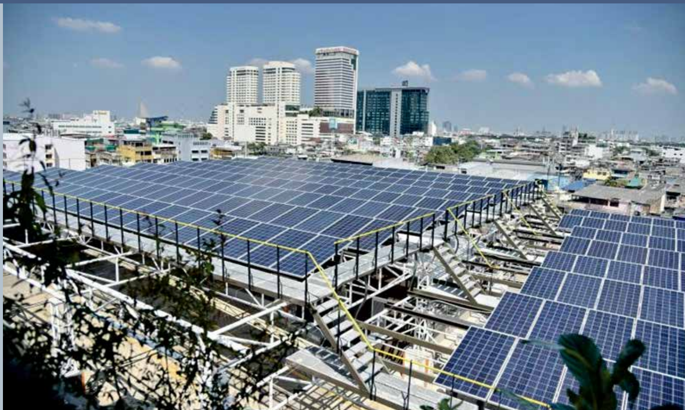
Fig. 1 – The 75 kW PV rooftop project installed over the parking building of the Department of Alternative Energy Development and Efficiency, Ministry of Energy of Thailand. The project aims to introduce demand-side management program to increase renewable energy consumption in the building using Building Energy Management System (BEMS) to balance between generated power and electricity demand, and to cut peak demand of building electricity need (Photo: DEDE).
