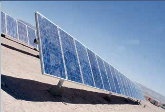
Fig. 1 - Calama Solar 3. The excellent local radiation conditions, in combination with the one-axis tracking systems, makes this 1 MW plant to deliver an outstanding annual generation of 2 900 MWh.
