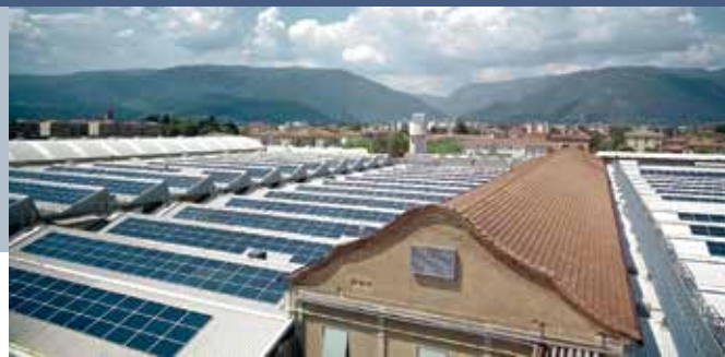
Fig. 4 – 1 MW PV plant on the BAXI roofs in Bassano del Grappa, which uses monocrystalline FU270P modules (Photo: FuturaSun).
