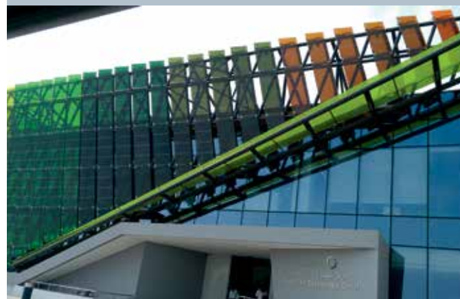
Fig. 6 - Construction work from ONYX SOLAR for the installation of BIPV in DEWA's building for R&D (Dubai).
