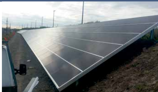
Fig. 1 - PV system for Øresundsbroen (the bridge between Denmark and Sweden). The power of the system is 255 kWp. System delivered by Helge Andersen, Solarpark DK A/S, Denmark.
