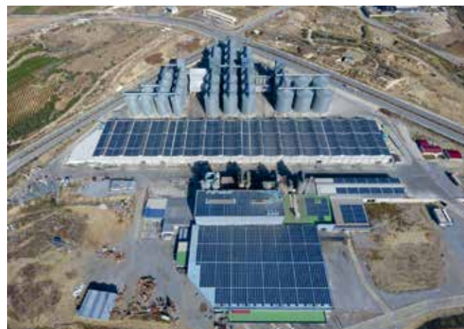
Fig. 2 - Commercial rooftop PV power system at Tiryaki Agro Company in Mersin (4.24 MW) [23].
