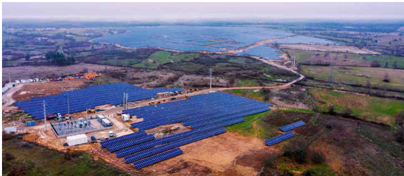
Fig. 1 - PV plant Mogadouro, in northern Portugal, with an installed peak power of 48,9 MW (Photo: Smartenergy).
