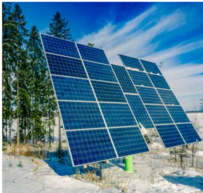
Fig. 1 - LUT two-axis tracking solar PV system (Photo: Teemu Leinonen).
