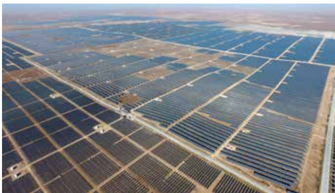
Fig. 4 - Ningxia 2 GW PV project (Photo: SUNGROW).
