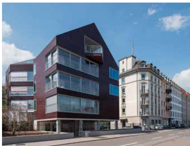
Fig. 3 - Complete BIPV building envelope at the Wohnhaus Solaris in Zürich by huggenbergerfries. Coloured modules from ertex solar (Photo: © ertex solar, Dieter Moor).
