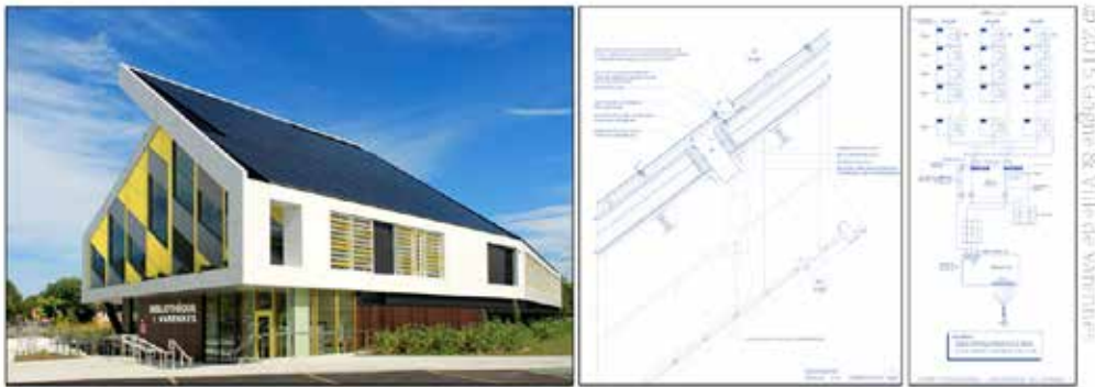
Fig. 2 - One of the selected BIPV projects analysed for the guidebook in preparation: BIPV roof at Varennes Library, Canada, and corresponding technical CAD drawings.
