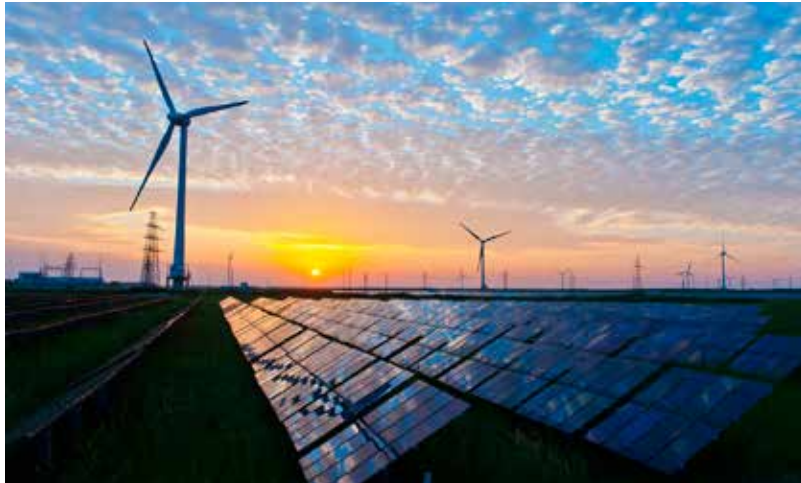
Fig. 1 - The main renewable electricity generation technologies require copper to operate. In a PV plant, copper is present in the conductive strips of cells and modules, in cables, inverters and transformers.
