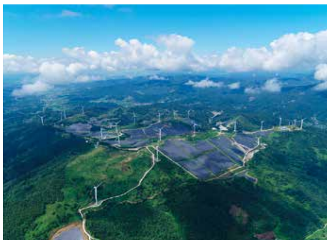
Fig. 2 - 94 MW PV system at Yeongam-gun, Jeollanam-do, Korea.
