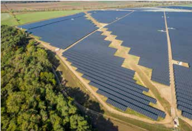
Fig. 2 - 187 MW commercial subsidy-free solar park in Weesow-Willmersdorf (Photo: © EnBW).
