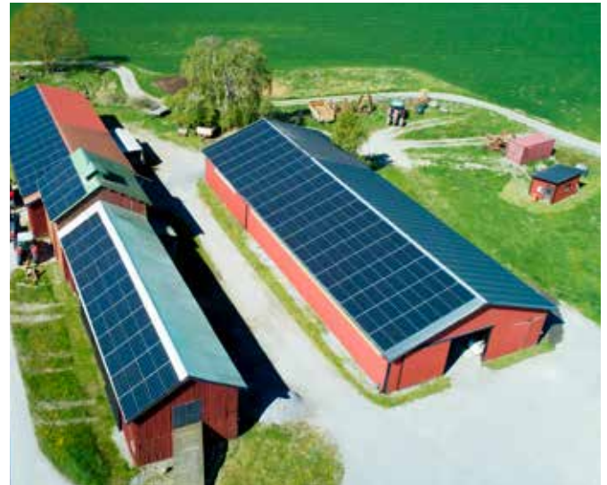
Fig. 3 - Example of a typical Swedish decentralized PV installation (Photo © HP SolarTech).
