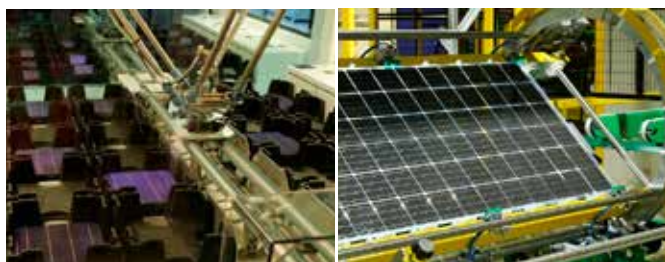
Fig. 6 - EGP 3SUN PV module factory: HJT bifacial cells' and modules' assembly lines (Photos: EGP).
