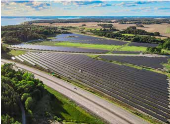
Fig. 1 - The largest PV plant in Sweden to date at 14 MWp. The plant lies outside of Strängnäs and was installed by EnergiEngagemang for HSB Sörmland (Photo: © EnergiEngagemang).
