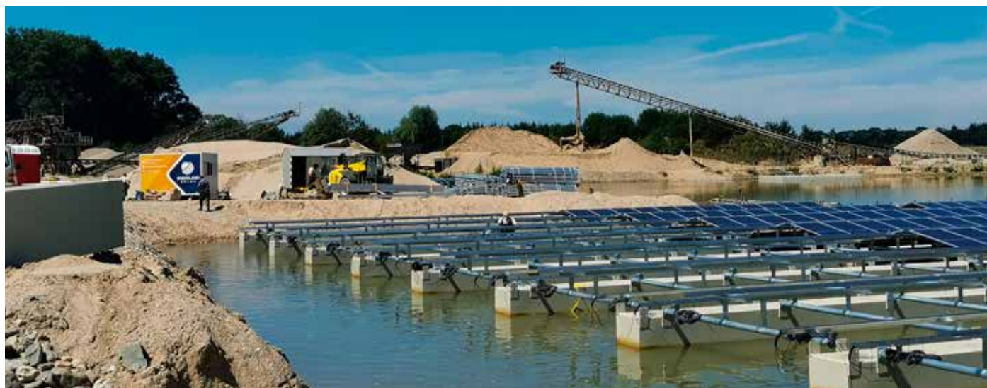
Fig. 6 - 750 kW floating PV on a dredging lake of a gravel pit (Photo: © Energieagentur.NRW / Rheinland Solar).
