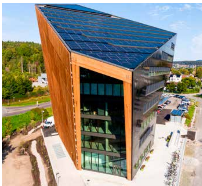
Fig. 1 - Powerhouse Telemark. This building's energy efficiency is due to a combination of architecture and technology. It has solar panels as façade and roof-top elements and uses innovative technologies for ventilation and heating (Photo: R8 Property/Tor Helge Thorsen).
