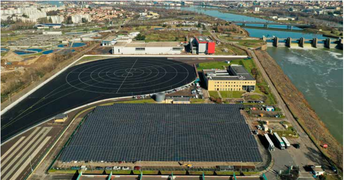
Fig. 1 - Solar parking canopies on the site of automotive industrial JTEKT Technical Center, in the Vallée de la Chimie near Lyon, France (Photo: Terre et Lac).
