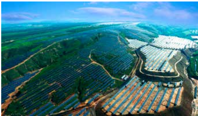
Fig. 3 - Baicheng PV Project (Photo: SUNGROW).
