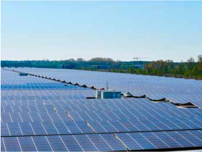
Fig. 2 - The biggest ground mounted PV power plant of Belgium (Lommel). The Kristal Solar Park - 99 MWp – was built in 2018-2019 and provides solar energy to the nearby zinc specialist company Nyrstar. This generates a yearly reduction of 30 000 tonnes of CO 2 (Photo: Engie).
