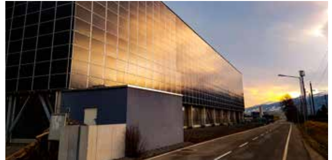
Fig. 2 - M Preis Supermarket's deep-freeze warehouse, Innsbruck, Austria. Winner of the 2 nd Austrian Award for building integrated PV for their complete energy concept including hydrogen (Photo: © ATB-Becker, Tyrol).
