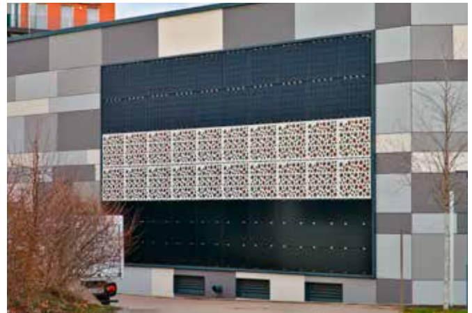
Fig. 3 - Demonstration BIPV façade at Fraunhofer ISE, Freiburg with CIGS (bottom), OPV (middle) and Silicon modules (top) (Photo: © FhG ISE).
