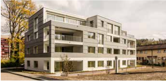
Fig. 1 - Multi-family house with PV façade; Winner of the 2 nd Austrian Award for building integrated PV (Photo: © Rene Schmid Architekten und Kioto Photo-voltaics).
