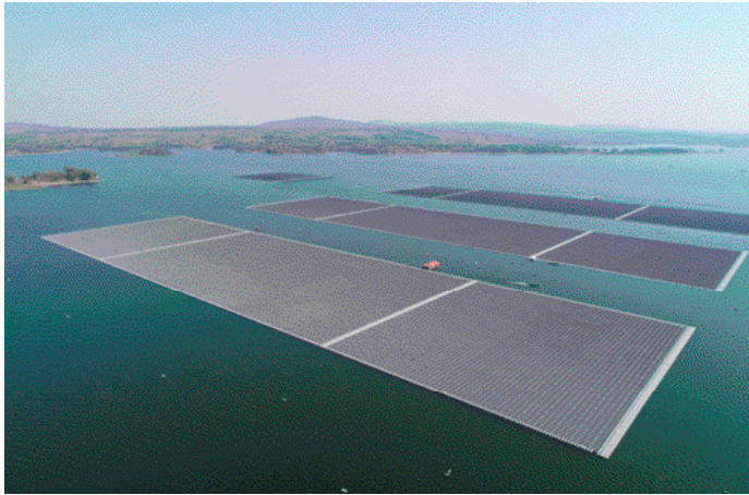
Fig. 1 - The 45 MW world's largest floating PV system, as part of the Hydro-Floating Solar Hybrid Project at Sirindhorn Dam, operated by the Electricity Generating Authority of Thailand (EGAT). This project will hybridize the FPVs with the hydropower dam to increase efficiency of the system (Photo: EGAT).
