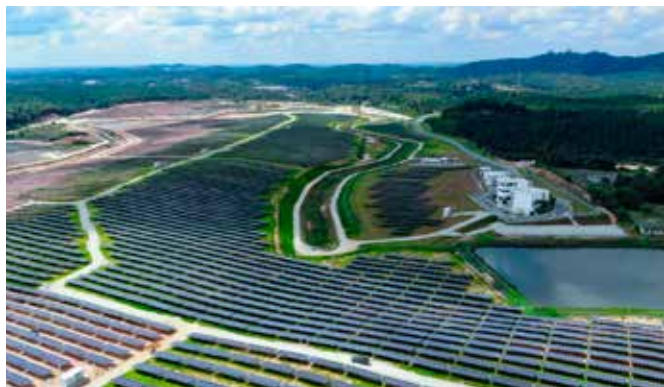
Fig. 1 - The 50 MW UiTM Solar Park I in Gambang, Pahang also houses a research centre on Renewable Energy, the first university in Malaysia to operate two LSS plants (Photo: UiTM Energy & Facilities Sdn. Bhd.).
