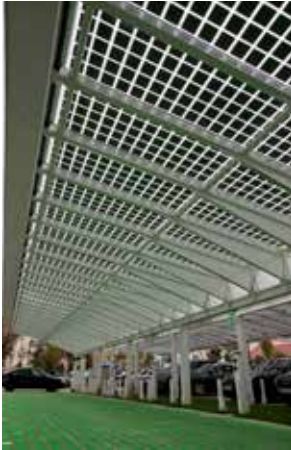
Fig. 3 - PV parking lot at the Arrival Center Schönbrunn (Photo: © ertex solar, Dieter Moor).
