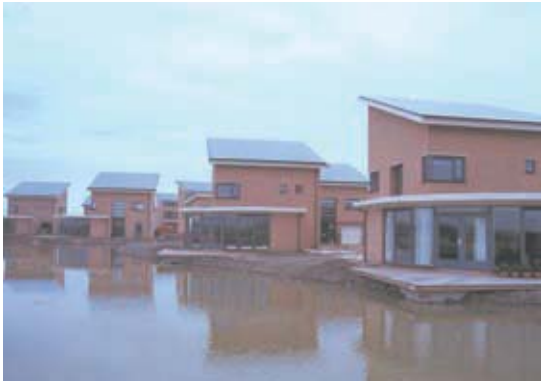
Figure 5: Langedijk solar and sustainable housing (some of the 2600 houses with 3775 kWp) in the Netherlands. Source: BEAR Architecten, photo: M. van Kerckhoven
