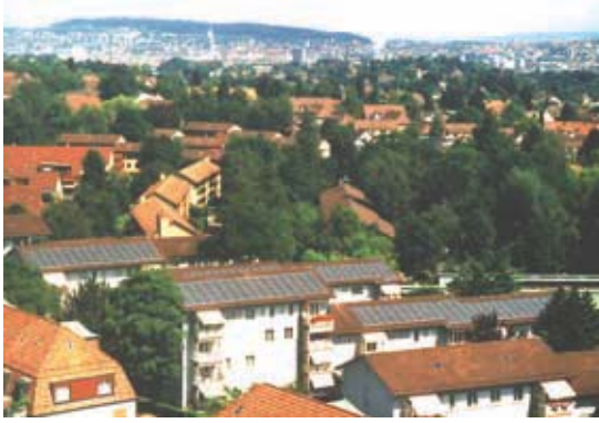
Figure 4: Marchwart project with roof integrated PV installation 53 kWp on multi-family buildings in a residential area of Zurich, Switzerland. Source: Enecolo
