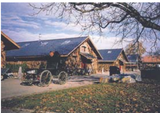
Figure 7: National equestrian centre in Bern, Switzerland, with four roof slopes fully covered with sunslates (80.5 kWp). Source: Atlantis Solar Systems
