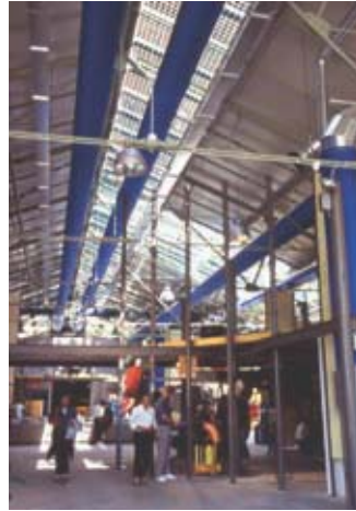
Figure 8: Children's Museum of Rome, Italy, with a semi-transparent canopy of 8.2 kWp solar power. Source: Abbate e Vigeveno Architetti
