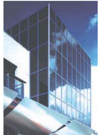
Figure 9: Industrial building with façade integrated PV system (8.4 kWp) at APS Photovoltaic Factory in Fairfield, California, USA. Source: DOE
