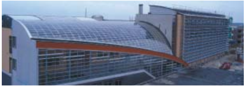
▲ Figure 6.4: ECN office and laboratory buildings. Architectural value for new and refurbished buildings - Images of the ECN office and laboratory buildings in an innovative design. Roof integrated PV system and refurbished façade with photovoltaic shading elements (102.9 kWp). Source: ECN, Petten, The Netherlands. Picture: M. Van Kerckhoven, BEAR Architecten, Gouda, The Netherlands.
