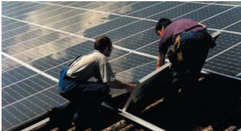
◀ Figure 2.1: To have a smooth procedure, photovoltaic integration should be considered from the very start of a project. Solar panels are mounted onto the roof in Hünenberg, Switzerland. Installed power is 32.56 kWp and produces solar electricity equivalent to the electricity consumption of 8 "average" Swiss families. Source: Urs Bühler, Cham, Switzerland.
