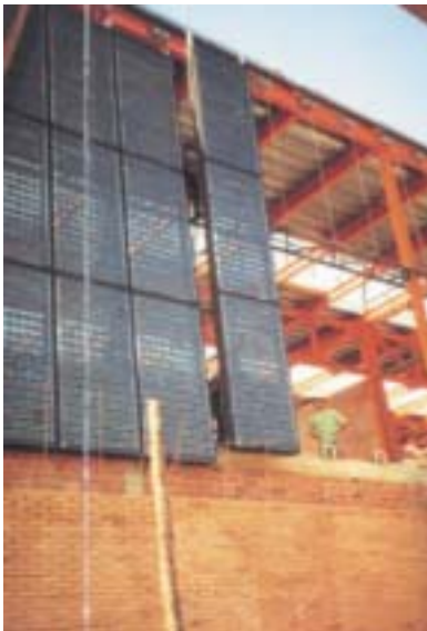
▲ Figure 1.3: Intelligent building design and construction process - mounting and integration of solar modules into the Mataró library building in Barcelona, Spain. The photovoltaic modules are at the same time façade elements and are part of the solar power station (53 kWp). Source: TFM, Spain.
