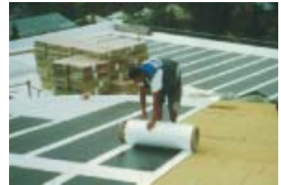
▲ Figure 6.12: Installation of solar membrane roof equals standard installation techniques. Source: Uni-Solar - Bekaert ECD Solar Systems LLC, Belgium; Picture: Alwitra GmbH, Germany.
