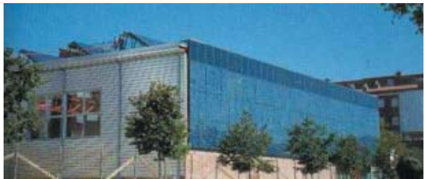
◀ Figure 6.1: Photovoltaic roof (Shopping centre entrance, Zurich, Switzerland). Here 30.5 kWp of photovoltaic cells are integrated into an atrium roof. The system is multifunctional - in addition to electricity it also provides optimum natural lighting levels, shading, weather protection and a suitable light reflection surface for night lighting. The installation was contracted by the Migros company as part of their corporate environmental policy. Power is sold via the innovative Solar Stock Exchange scheme of the local electricity utility (See the following chapter for further details). Source: energiebüro® Zurich, Switzerland.
