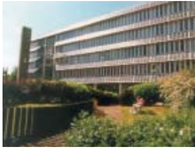
▲ Figure 6.3: University of Northumbria, UK. This 39.5 kWp installation is the result of a refurbishment project at the University of Northumbria in Newcastle. Photovoltaic panels have been incorporated into the new over-cladding of the building and the electricity produced contributes to meeting the building's needs for lighting, computers and other appliances. Any surplus electricity can be fed into the University's internal distribution system to supply other buildings on the campus. Source: Tymandra Bewett-Silcock.
