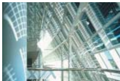
◀ Figure 5.4 a+b: Photovoltaics incorporated as shading elements – building for the University of Erlangen, Germany (a) vs. semi-transparent photovoltaics – Doxford office building, UK (b). Source: (a) Solon AG, Berlin, Germany. (b) Studio E. Architects, London, UK.
