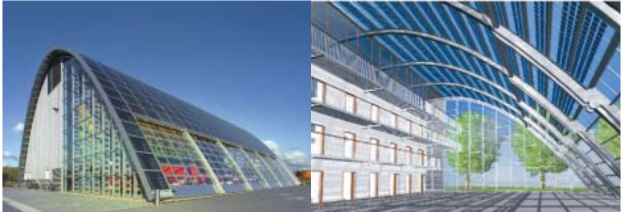
▲ Figure 2.3 a+b: Fire Station Houten (Netherlands), 400m 2 photovoltaic (transparent), 24 kWp, 18000 kWh per year (10% of total electricity use). Architect: Samyn & Partners, picture by Richard Schropp.
