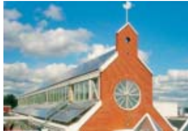
◀ Figure 5.13b: Combining photovoltaic integration and respect for traditional building styles in new construction is possible as this example clearly shows. (Lieliahti Citymarket in Tampere, Southern Finland), Source: Naps Systems Oy.
