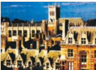
▲ Figure 5.11: Listed buildings and conservation areas present a challenge for BIPV potential (Cambridge, UK).
