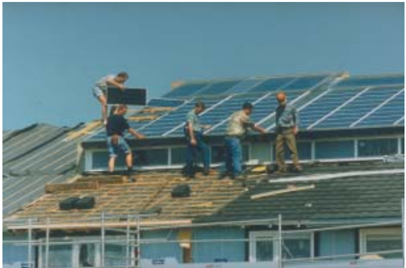
▲ Figure 0.2: Roof to be clad and turned into a multifunctional building skin. Source: Ecofys, The Netherlands.
