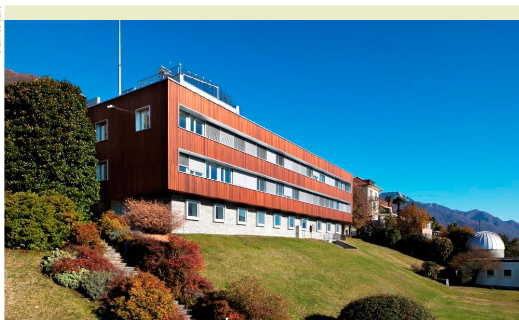
The MeteoSwiss building in Locarno Monti was renovated in 2012. The existing oil heating system and cooling equipment were replaced with a heat pump system with geothermal sensors. In addition, a photovoltaic system with an output of 20 kWp was installed.
