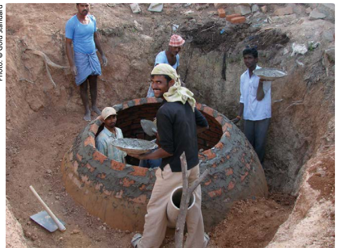
Construction of a micro-biogas plant in one of the selected compensation projects.
