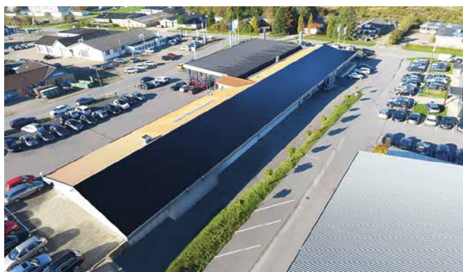
Fig. 2 – 31 kW Ennogie Solar Roof on Automobile Shop. The sales and display area of the company has large window areas and heat from the sun is a problem in the summer. To accommodate this, the owner has several air conditioning units installed which use a lot of electricity. Since the AC is needed when the sun is shining, it matches the production from the roof very well. With the Ennogie Solar Roof, the AC basically runs for free and saves the customer expensive grid electricity. ROI is less than 4 years.
