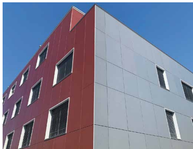
Fig. 3 – Plus energy multi-family house completed in 2019, with an active solar façade (glass/glass with monocrystalline cells). The total PV surface is 690 m 2 with a nominal power of 65 kWp. Final yield: 385 kWh/kWp. The ventilated construction was pre-assembled in the factory, avoiding the need to measure and set the substructure on the building. The whole installation was greatly simplified (Photo: © Viridén + Partner AG).
