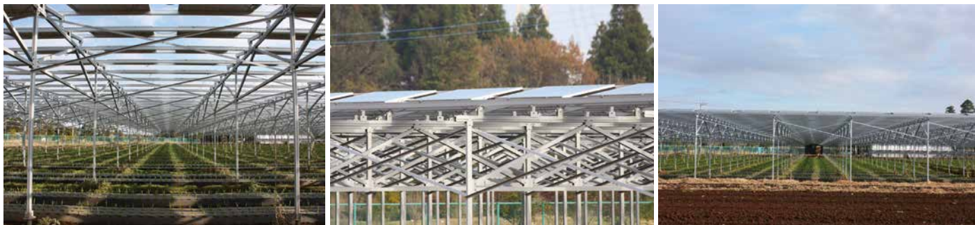
Fig. 2 – PV Systems on farmland (Chiba City Okido Agri Energy Unit 1) (Midori Ward, Chiba City, Chiba Prefecture). Installed capacity: 777,15 kWDC.
