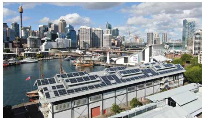
Fig. 3 – Flexible, light-weight PV Module installation on the Sydney Maritime Museum. Modules by Sunman (Photo: Energen Pty Ltd.).
