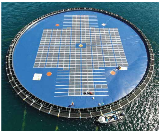
Fig. 1 – Flexible floating structure with PV modules (Source: Børge Bjørneklett, Ocean Sun).
