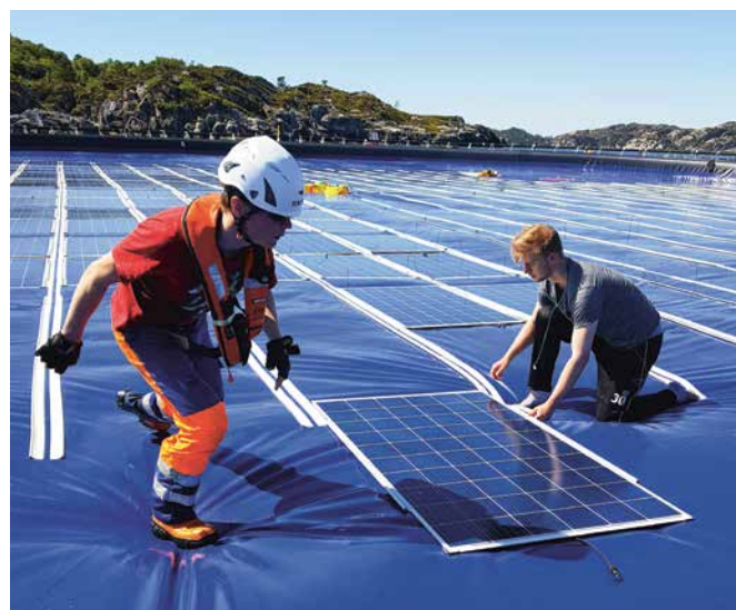
Fig. 2 – Installation of PV panels on the flexible floating structure (Source: Børge Bjørneklett, Ocean Sun).
