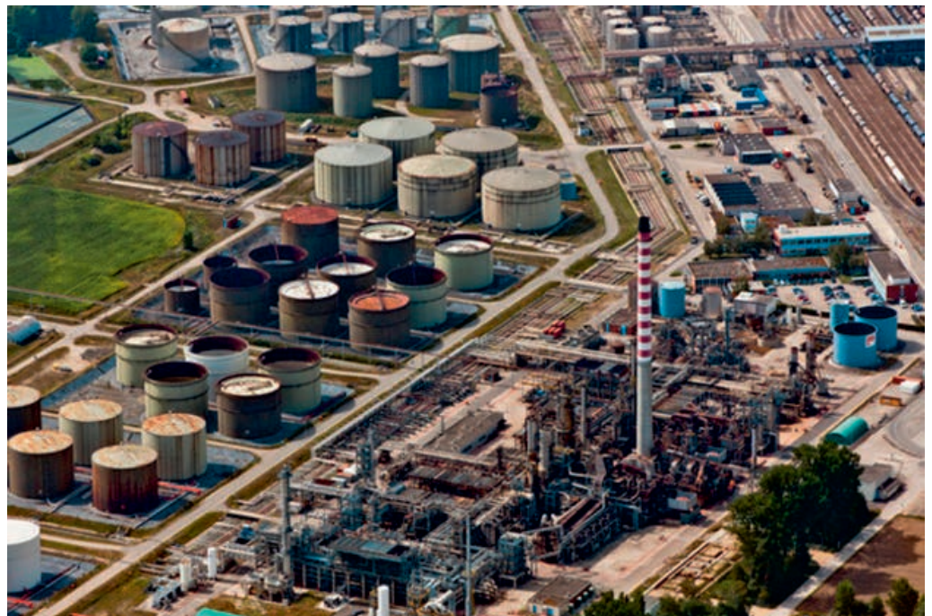
Raffinerie in Cressier (NE)
