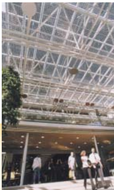
◀ Figure 6.1: Photovoltaic roof (Shopping centre entrance, Zurich, Switzerland). Here 30.5 kWp of photovoltaic cells are integrated into an atrium roof. The system is multifunctional - in addition to electricity it also provides optimum natural lighting levels, shading, weather protection and a suitable light reflection surface for night lighting. The installation was contracted by the Migros company as part of their corporate environmental policy. Power is sold via the innovative Solar Stock Exchange scheme of the local electricity utility (See the following chapter for further details). Source: energiebüro® Zurich, Switzerland.
