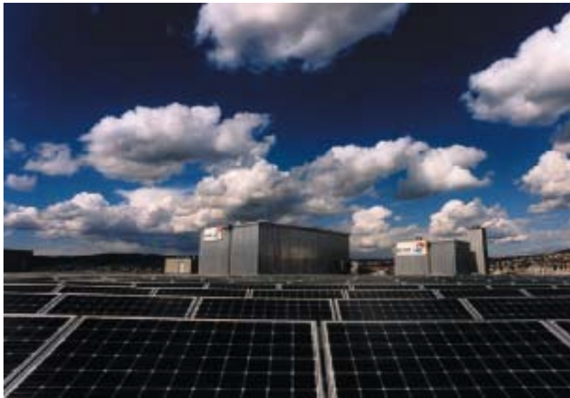
◀ Figure 1.2: Flat roof integrated photovoltaic installation with solar power of 270 kWp feeding the grid in Zurich. Copyright: Zollfreilager, Switzerland.
