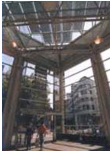
◀ Figure 7.9: Migros Limmatplatz Solar Power Station in Zurich, Switzerland. Installed capacity: 30 kWp. Energy production: 24000 kWh/yr. Photovoltaics surface: 360 m². Investment cost: 190000 €. Financing: Solar Stock Exchange. Source: energiebüro ®, Zurich, Switzerland.
