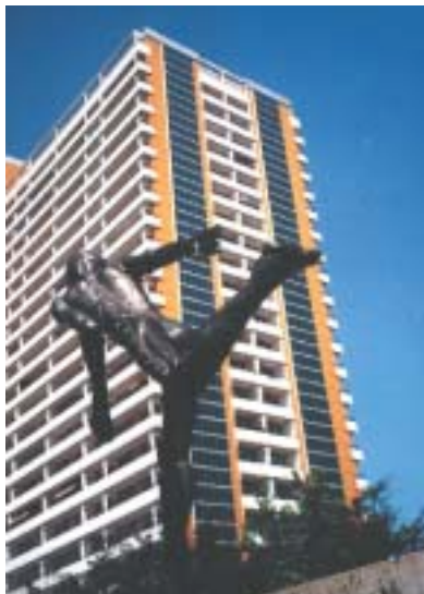
▲ Figure 0.1: Solar power in a refurbished façade in Berlin - Marzahn - Germany. Source: NET Ltd, St. Ursen, Switzerland.
