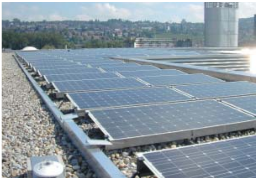
▲ Figure 2.3 a+b: Fire Station Houten (Netherlands), 400m 2 photovoltaic (transparent), 24 kWp, 18000 kWh per year (10% of total electricity use). Architect: Samyn & Partners, picture by Richard Schropp.
