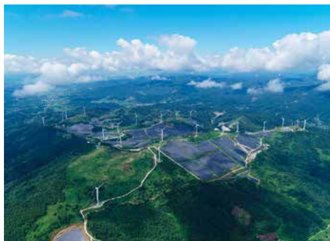
Fig. 2 - 94 MW PV system at Yeongam-gun, Jeollanam-do, Korea.
