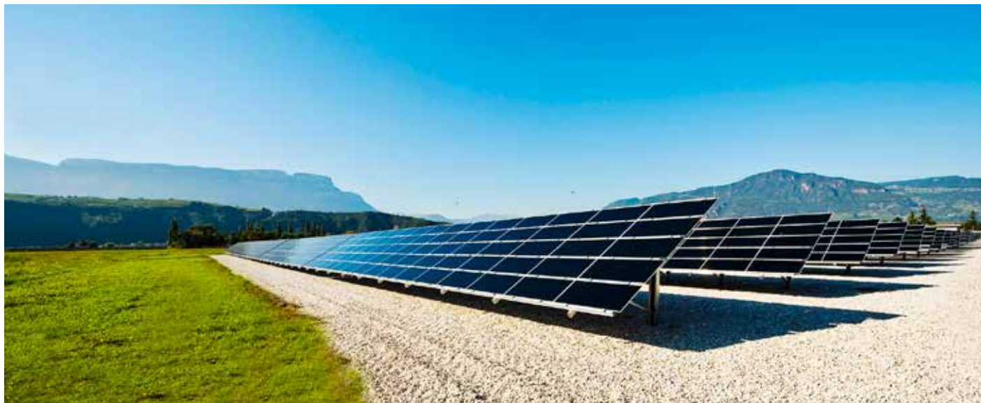
Fig. 1 - A multi-technology photovoltaic test facility for the detailed performance evaluation of different module technologies and mounting systems was set up by EURAC research in cooperation with Airport of Bolzano Dolomiti (ABD). It is operating since 2010 (Photo: EURAC /Othmar Seehauser).
