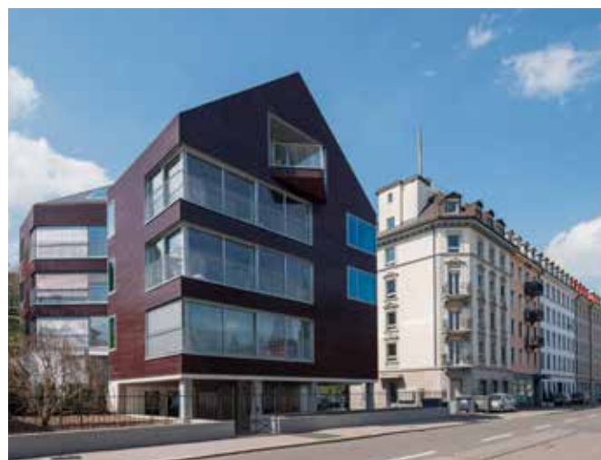
Fig. 3 – Complete BIPV building envelope at the Wohnhaus Solaris in Zürich by huggenbergerfries. Coloured modules from ertex solar (Photo: © ertex solar, Dieter Moor).
