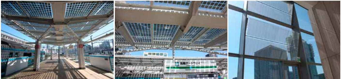
Fig. 1 - Roof and Window Glass-integrated PV System at Station Platform (Takanawa Gateway Station PV System) (Minato Ward, Tokyo). Power generation capacity: 43.8 kW (roof of platform), 1.1 kW (window glass). PV modules: Bifacial single-crystalline silicon PV modules (SUNJOULE® glass-integrated PV modules by AGC).
