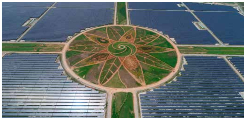
Fig. 1 – 98 MW PV system at Haenam-gun, Jeollanam-do, Korea.
