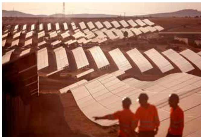
Fig. 7a - Construction of "Nuñez de Balboa" PV plant (500 MW in Badajoz, Spain) by the Spanish utility IBERDROLA.
