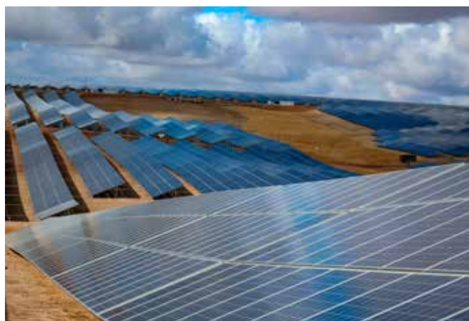
Fig. 7b - Completed construction of "Nuñez de Balboa" PV plant (500 MW in Badajoz, Spain), by the Spanish utility IBERDROLA.
