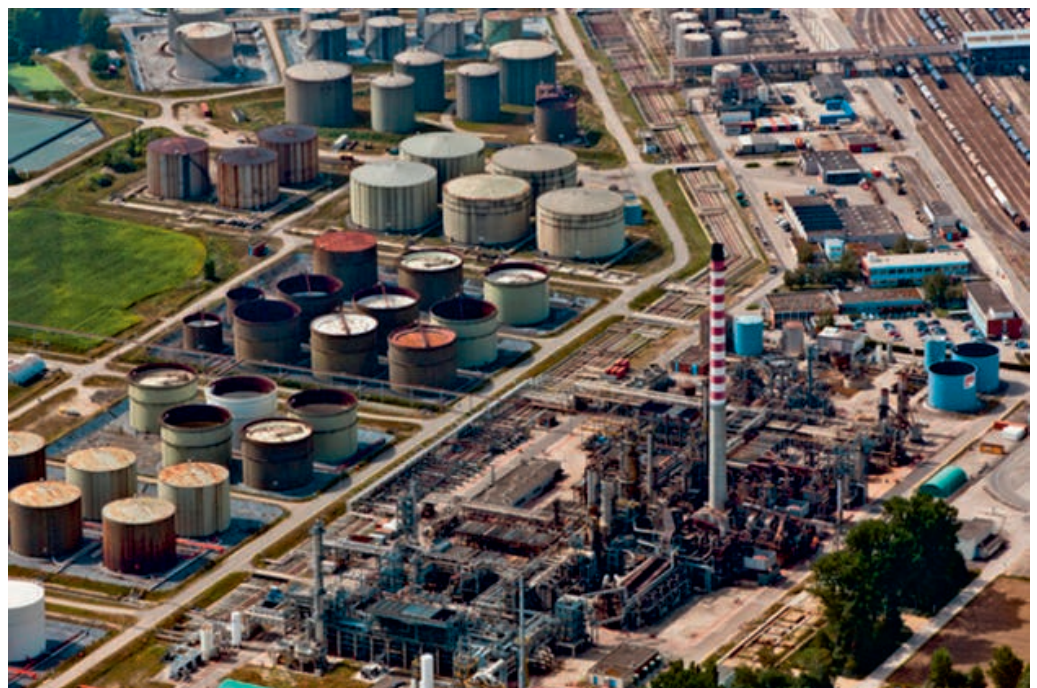
Raffinerie in Cressier (NE)
